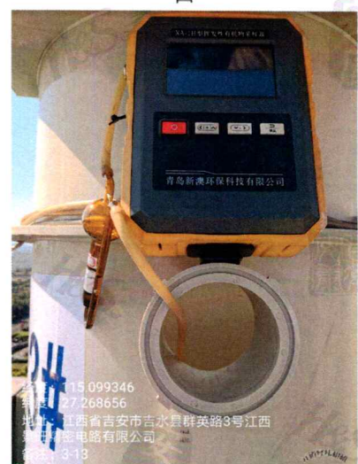
3-13#外层蚀刻废气排放口
