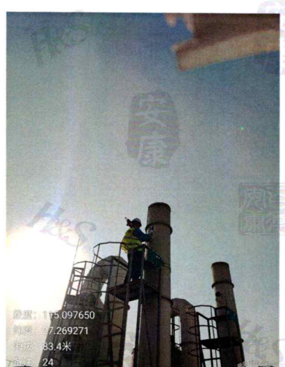
2-24#防焊前处理废气排放口
